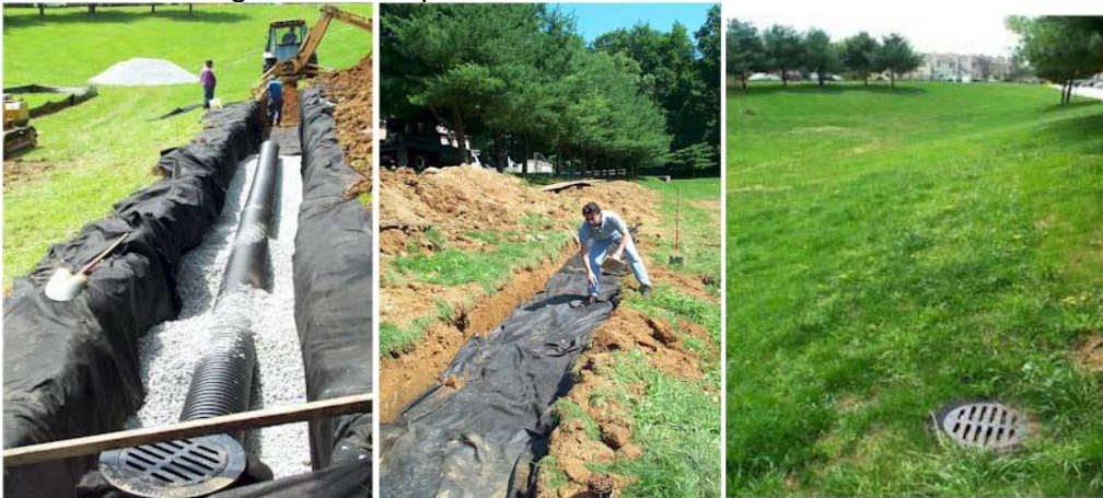
Figure 3: Example of Infiltration Trench Installation
