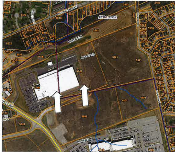
Springdale Avenue; Aerial photo showing proposed street vacation
