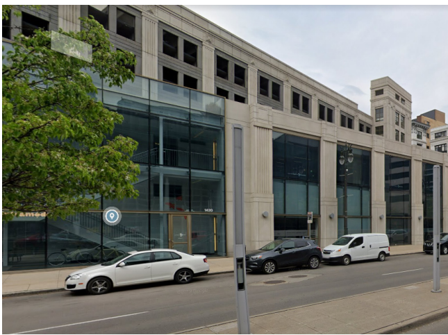
Parking Structures with Ground Floor Liner Buildings and screening for upper stories.
