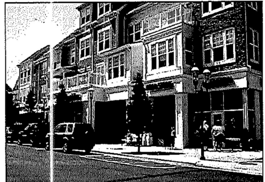
Image 2. Mixed use building with retail and residential
