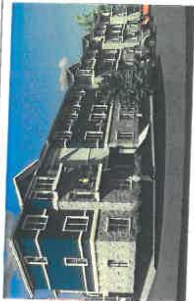
Exhibit C Proposed Roof Plan Modification Modified pitch to remove majority of flat roof area on 3-story portion of facility. Flat roof area will not be visible from grade.
