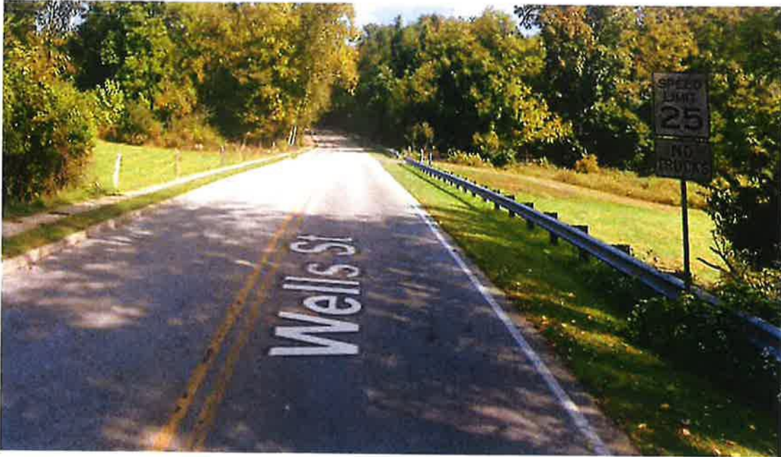
Figure 1 Speed Limit Sign on Wells needs to be replaced
