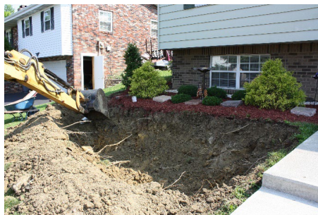
Excavate rain garden at least 10' from foundation
