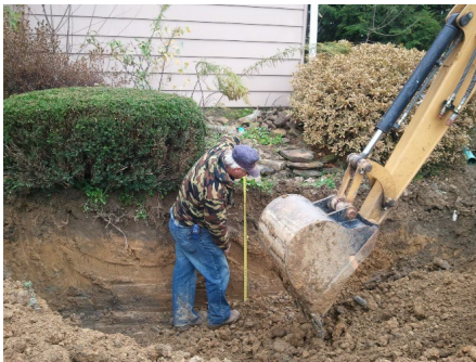
Excavate a drywell at least 10' from foundation
