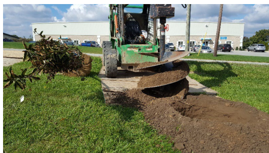
Plywood sheets protect lawn from compaction
