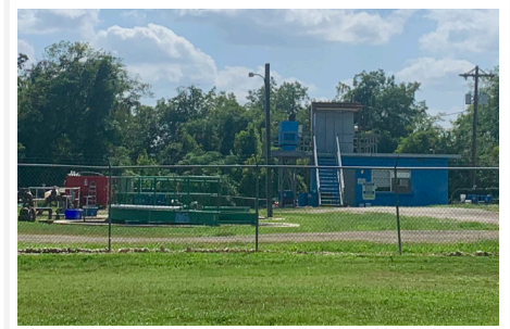
Bandera's Wastewater Treatment Plant. Bandera, TX 2021.
