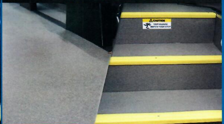
Flooring is a non-slip, commercial grade; Includes yellow step nosing; provides greater visibility for senior adults
