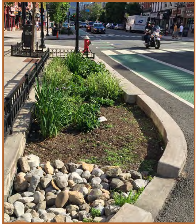
Rain gardens on public streets can manage stormwater, beautify the City, and calm traffic.
