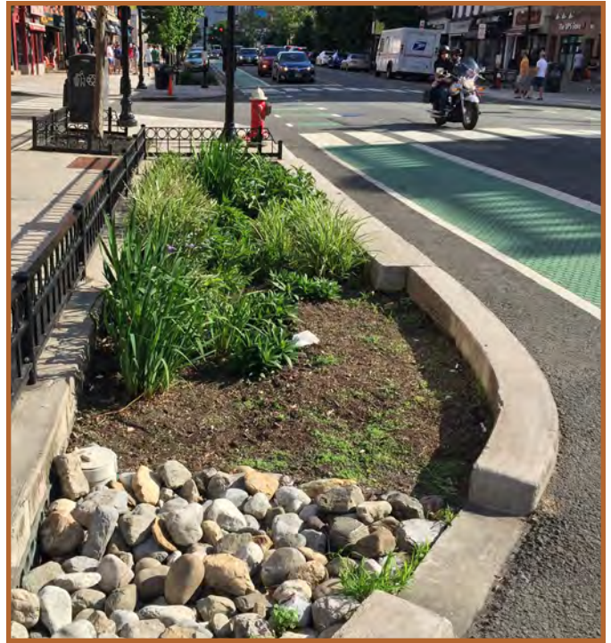
Rain gardens on public streets can manage stormwater, beautify the City, and calm traffic.
