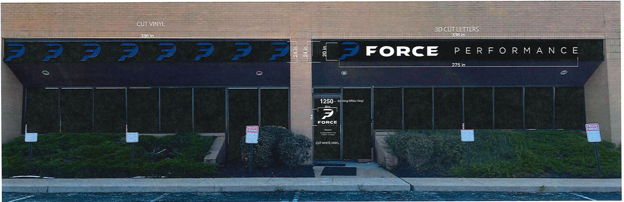
Force performance Building signs 8-13-21
