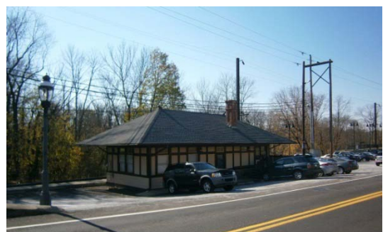
Chalfont SEPTA Station Source: Delta Development Group, inc.
