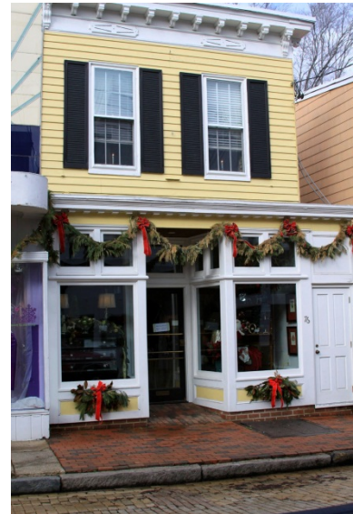
Historic Retail Façade in Annapolis, Md Source: Delta Development Group, Inc.
