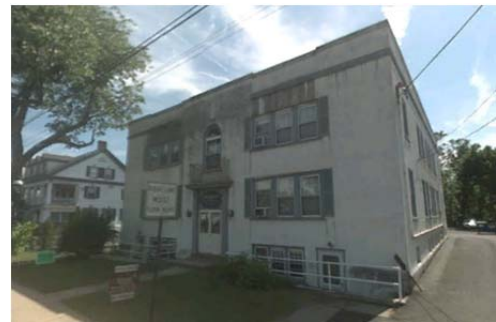
Existing Chalfont Plaza Source: Delta Development Group, Inc.
