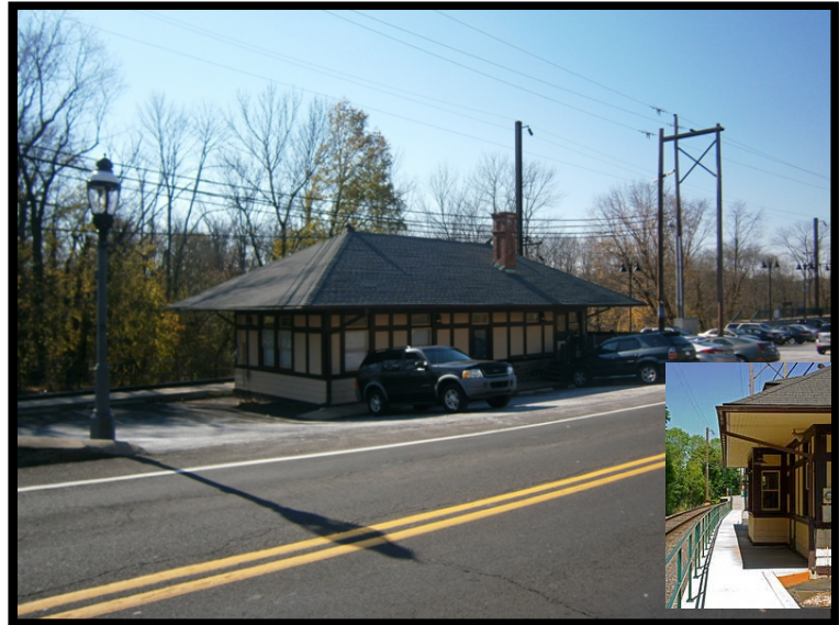
Chalfont SEPTA Station Source: Delta Development Group, Inc.
