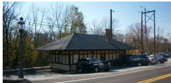
Septa Train Station Source: Delta Development Group, Inc.
