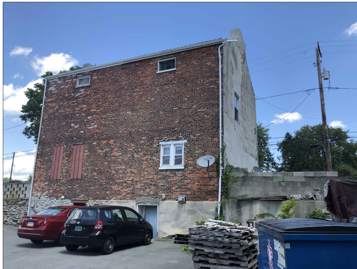
View from Southwest
