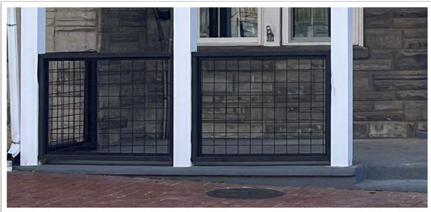
Figure 3- New Porch Railing Materials, October 2023 Columbia Borough Staff.
