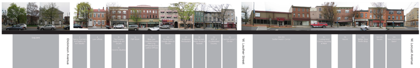
North Hanover Street Corridor - West Side Building Facades
