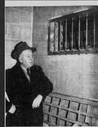
COLUMBIA POLICE CHIEF INSPECTS REPLACEMENT—Eugene M. McManus, Columbia police chief, looks over the iron bars installed in the borough jail window formerly covered with heavy screen mesh. The replacement was made after the escape Thursday of Clarence Price, 36, 115 S. 5th St., Columbia, who was being held for questioning in the theft of a parking meter last week from S. Fourth St., Columbia.
