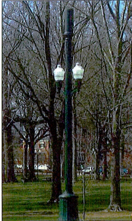
Extension of Existing Street Light
