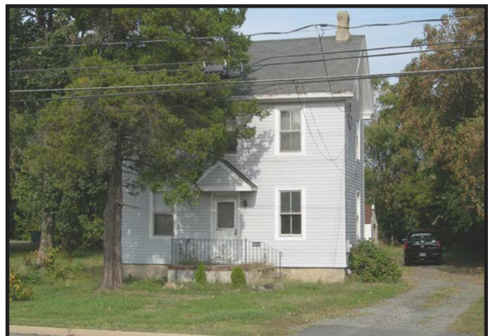
Off-Street Parking to the Rear of Building
