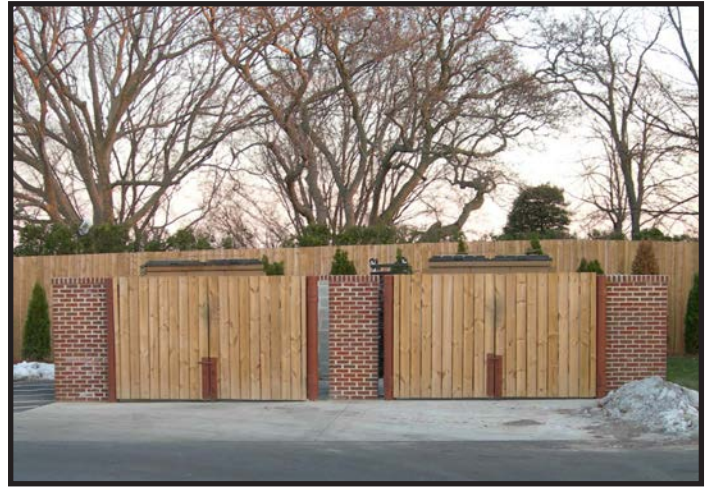
Architecturally Screened Dumpster
