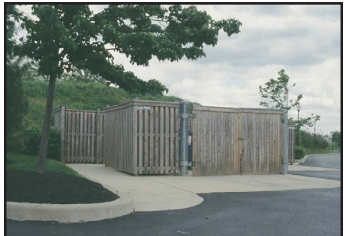
Dumpster Enclosure: Springhouse at Thornbury
