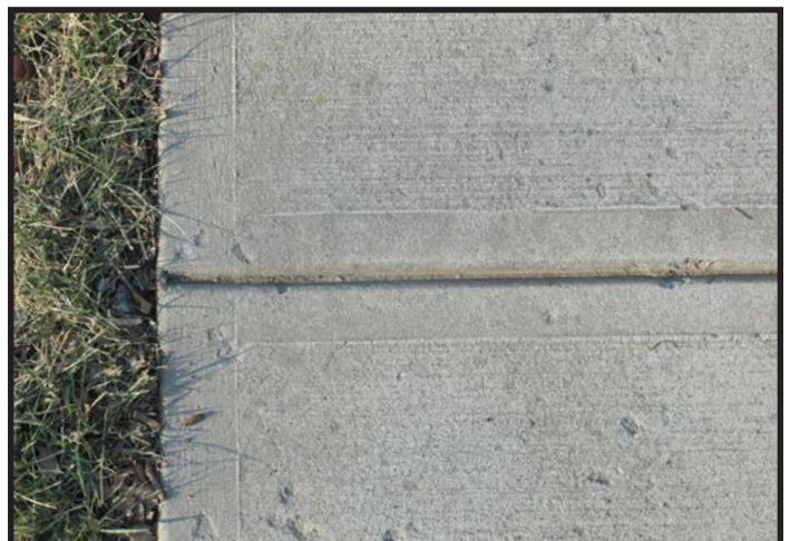
Concrete Pavement: West Chester, PA
