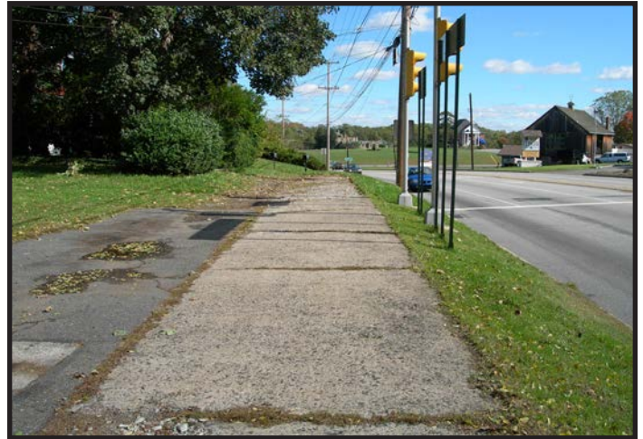
Existing Sidewalk in center of Concordville
