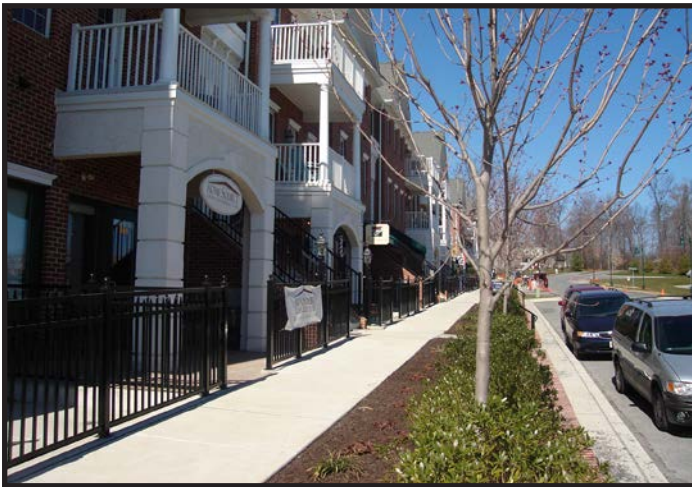
Example of Live-Work Units, Eagleview - Lionville, PA
