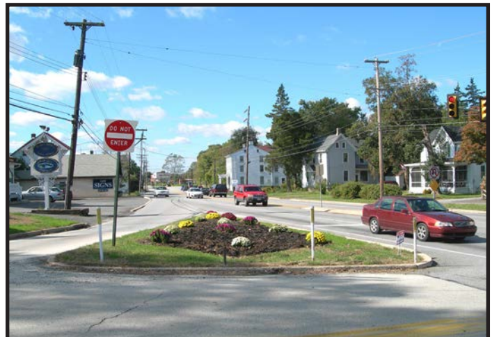
Landscaped Island as a Traffic Calming Measure
