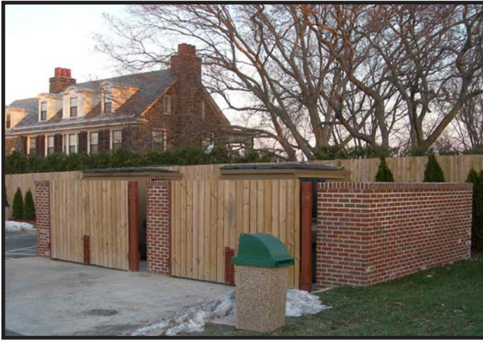
Brick Wall Enclosures of Dumpster
