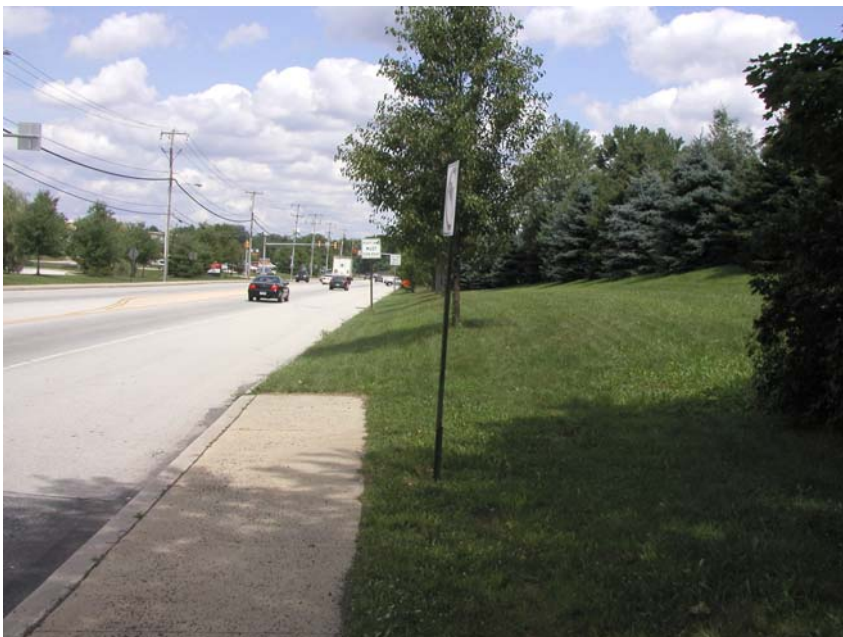
A need exists to complete the borough’s sidewalk network
