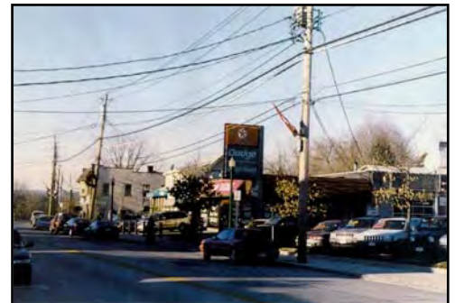
Overhead utility wires mar the streetscape along South Riverside Avenue.
