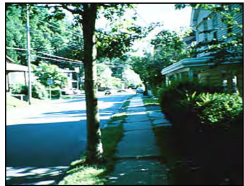
Sidewalk condition, Upper Village
