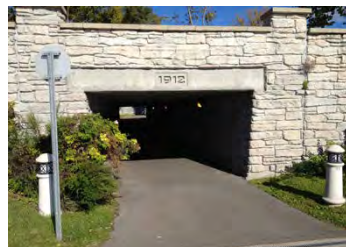
8: Senasqua Tunnel (pedestrian underpass to Municipal Pl.)
