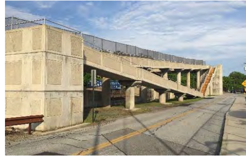
Brook Street Pedestrian Bridge
