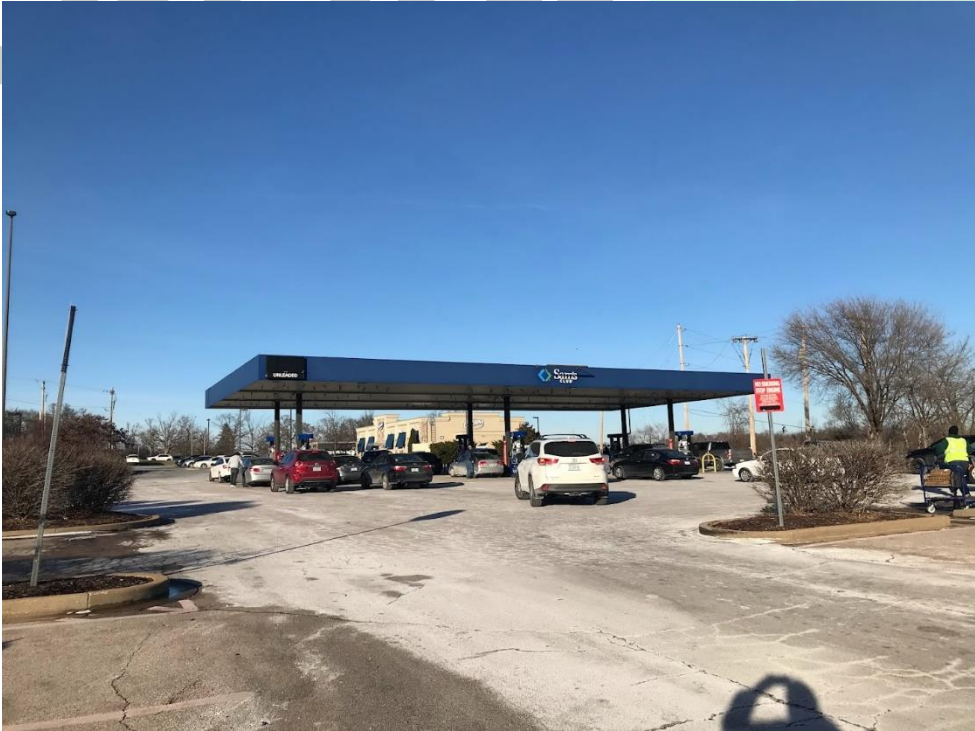
View from the south
