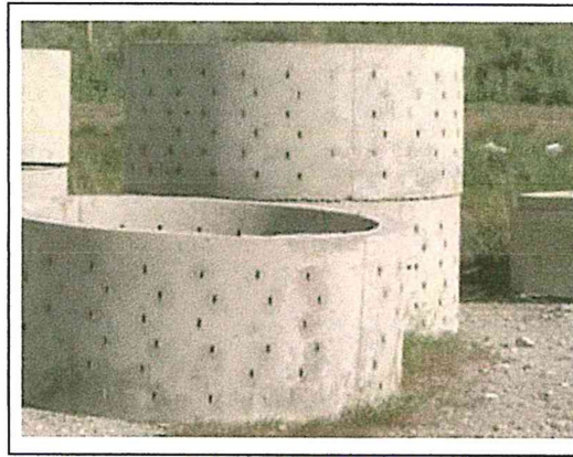
Figure E.4. Dry Well #1 – Structural Prefabricated Chamber.
