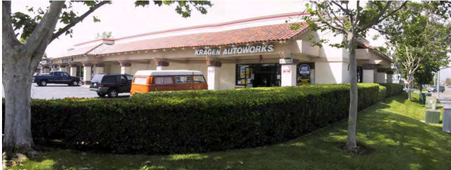
Covered arcades, heavy columns, stucco walls, tile roofs and rafter tails characterize the Mission style, commonly found along the parkway
