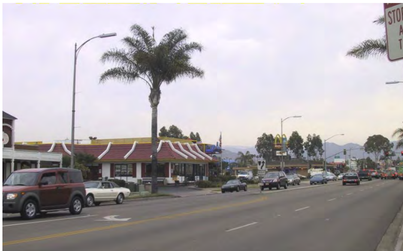
Mid-block left turn lanes, which facilitate access to individual businesses, may impede traffic flow
