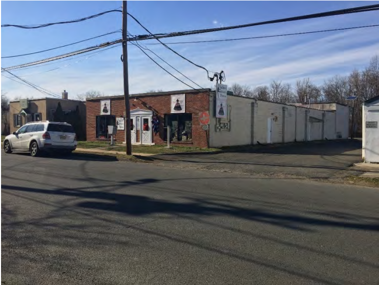
Commercial building as viewed from Lexington Ave. Photo taken February 2020
