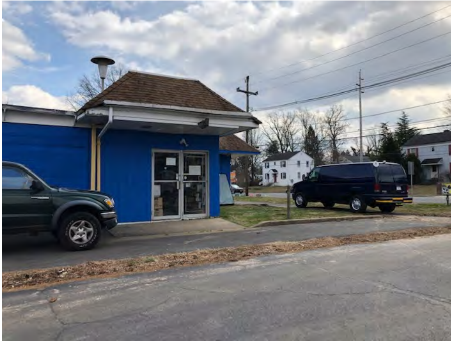
1960 N Olden Ave from Olden Avenue. View from N.Olden west side. Vehicles illegally parked on lawn. No vehicular or formal pedestrian access on this side of building. Photo taken February 2020
