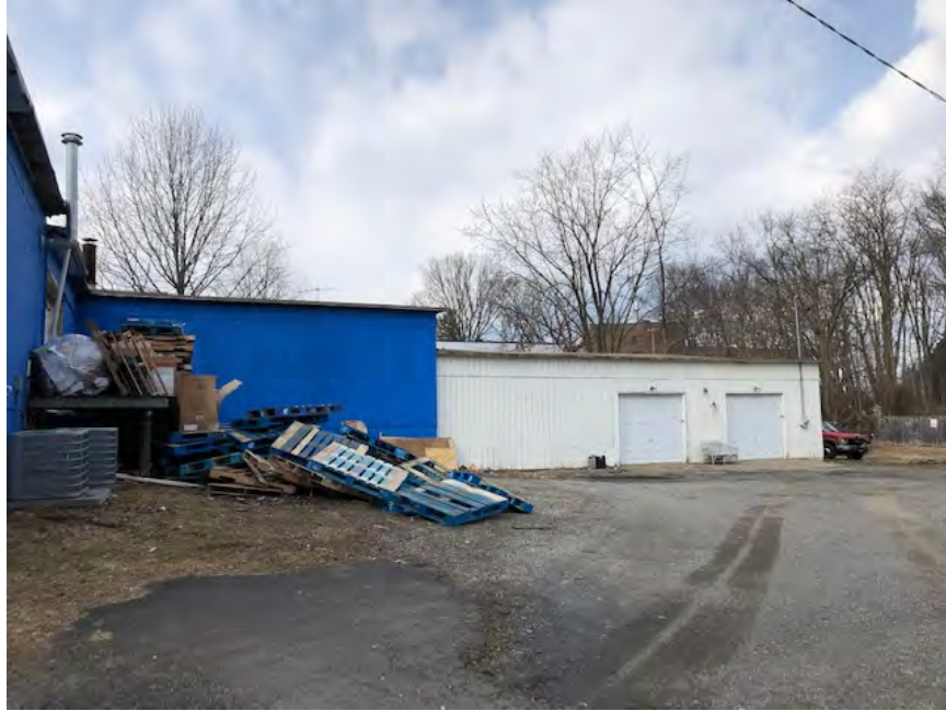
1960 N Olden Ave from Olden Avenue. Garbage violations. No use currently permitted in this section of building. Photo taken February 2020
