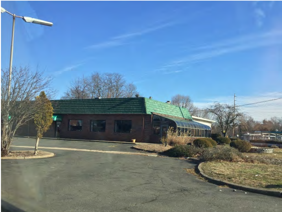
836 Parkway Ave from Parkway Avenue entrance. Photo taken February 2020.
