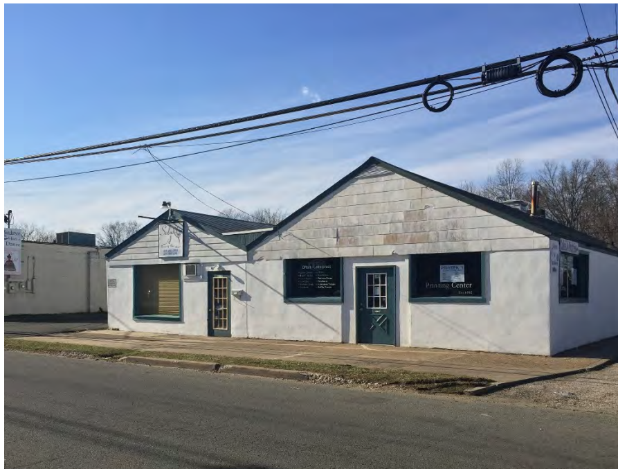
Commercial structure at 831 Parkway from Lexington Ave. Photo taken February 2020.
