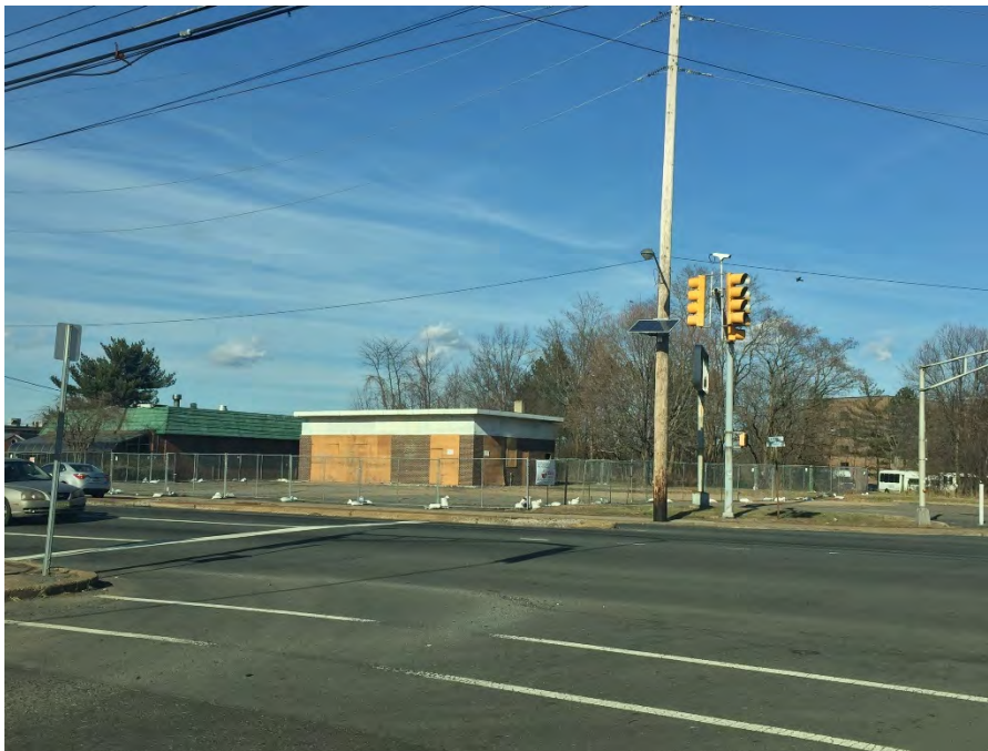
824 Parkway from the intersection of Parkway and Olden. Photo taken February 2020.
