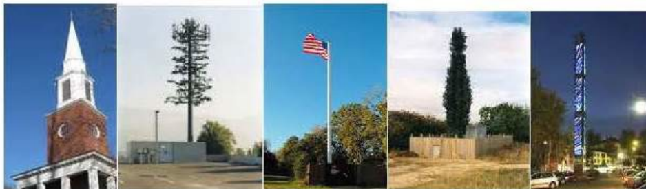
Figure 04.03-3 Examples of Concealed Facilities
