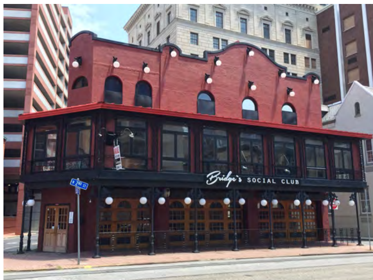
Although severely altered, the original Methodist Church and Ohev Sholom Temple on North 2nd Street was constructed in 1820. The building maintains its original stucco exterior.
