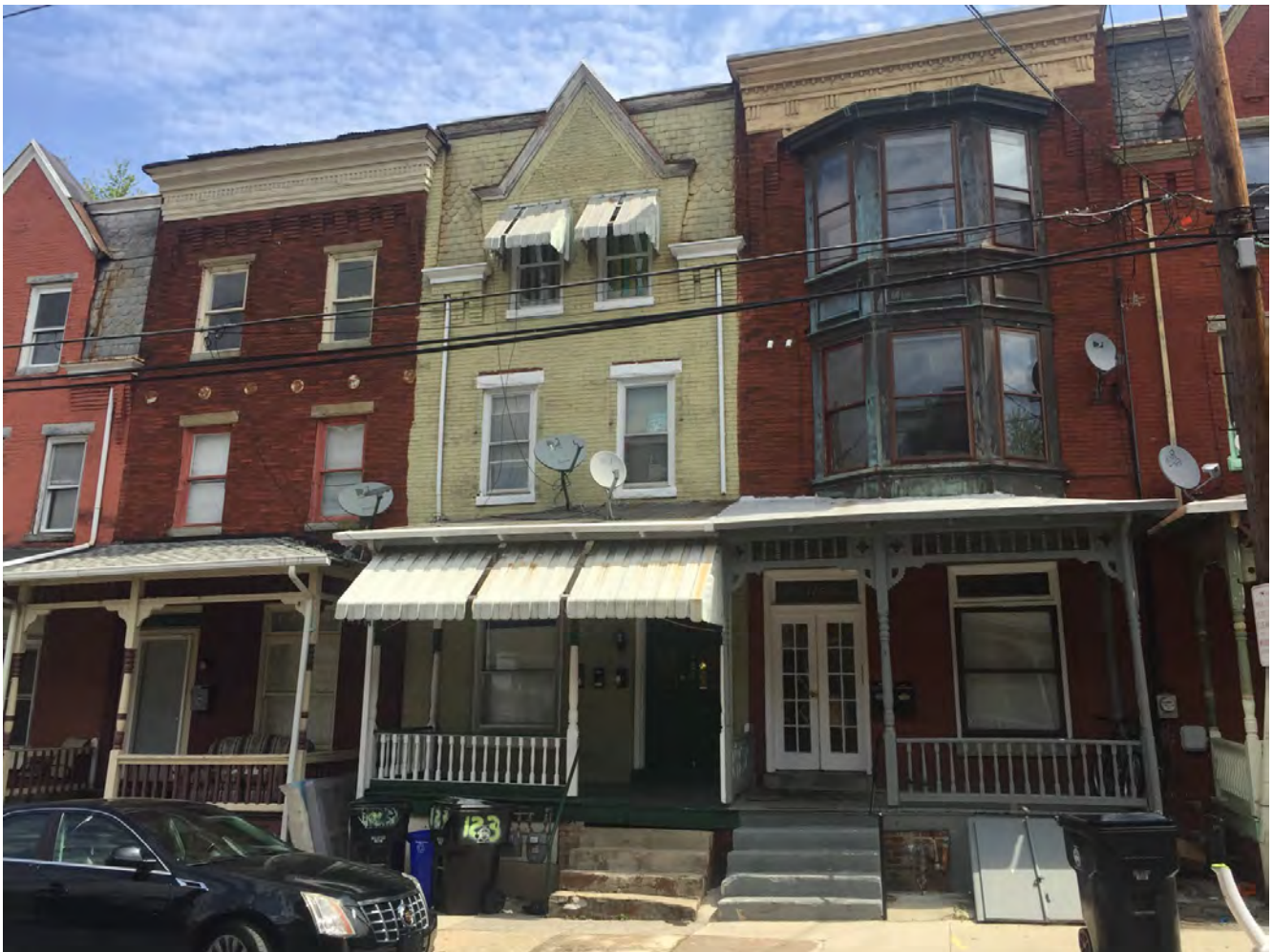
This historic streetscape is diminished by the installation of several satellite dishes. Such utilities should not be mounted on primary facades.
