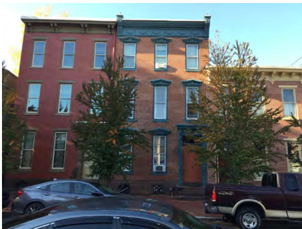
Example of Primary Facades
