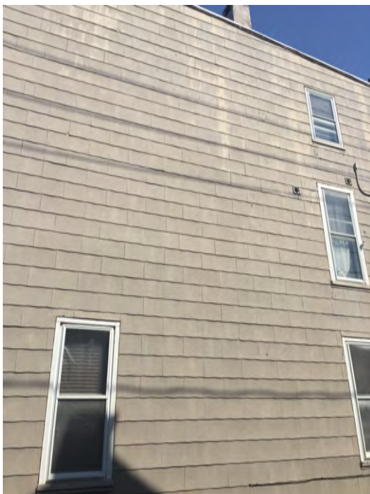
Asbestos-Cement shingles are long lasting and durable. Preservation treatments for this material depend upon the context of the building.
