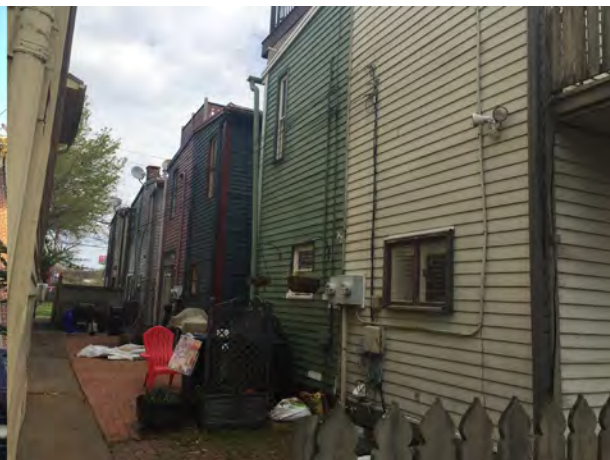
Example of Secondary Facades
