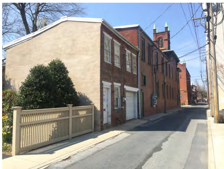
An example of a stucco party wall in Midtown. These walls can be repaired and maintained as needed.
