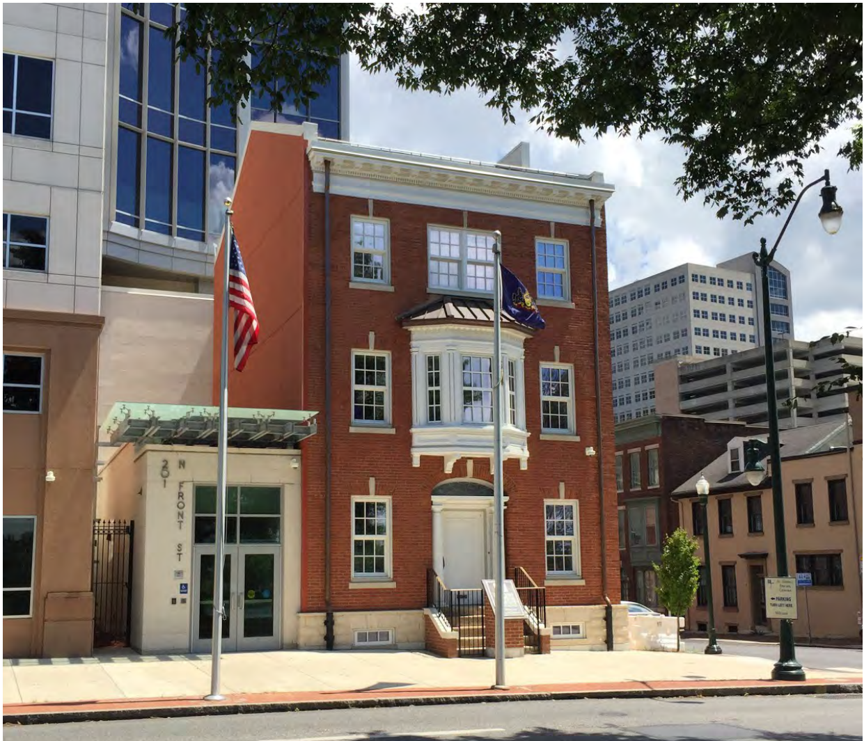
The Hickok Mansion on North Front Street was rehabilitated and required a new addition for continued use. The small addition to the left of the mansion is a compatible yet subordinate to the historic building.
