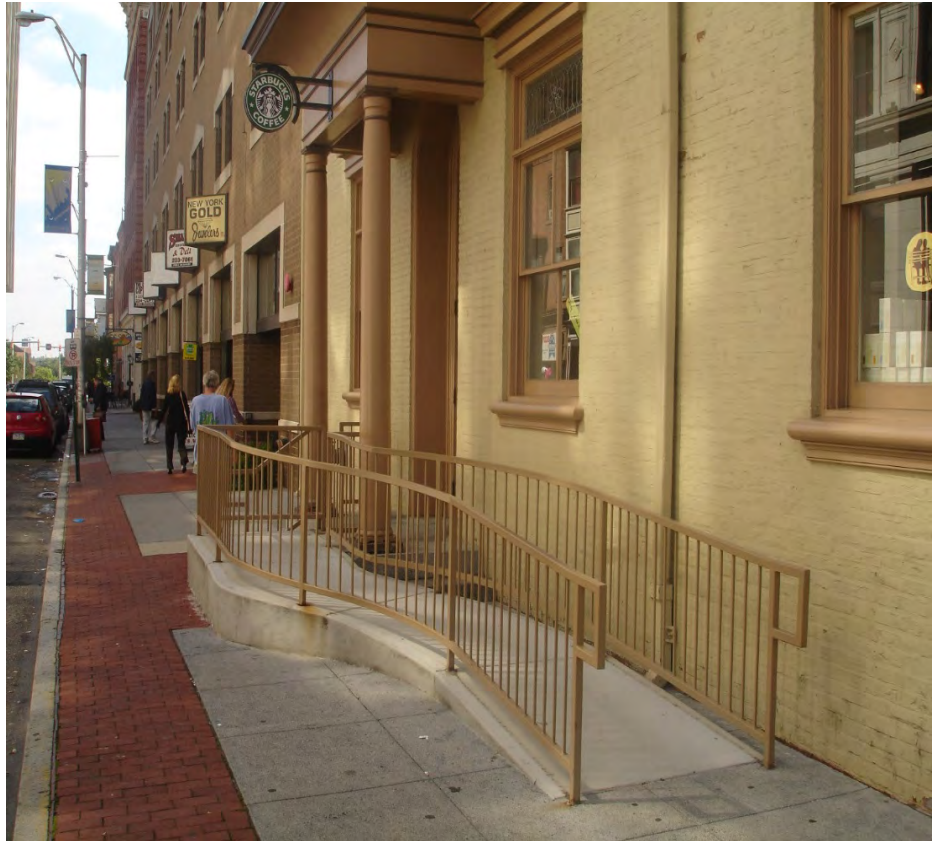
This ramp was installed on a secondary facade and it blends in with the historic neighborhood without causing any adverse effects on historic materials.
