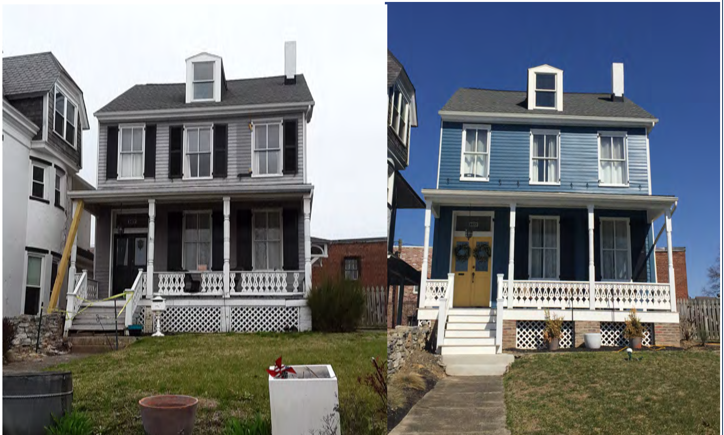
This historic Front Street residence has undergone extensive rehabilitation to its exterior including a porch restoration and a fresh paint job.
