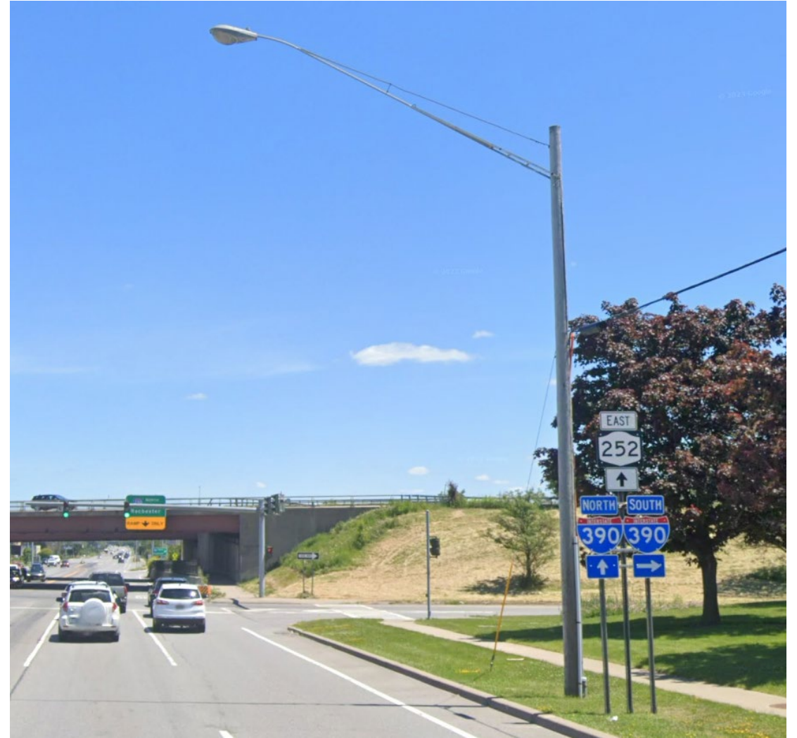
Pole in front of 1111 Jefferson Rd
