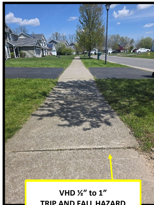
VHD ½" to 1" TRIP AND FALL HAZARD Repairable using Precision Concrete Cutting Process
