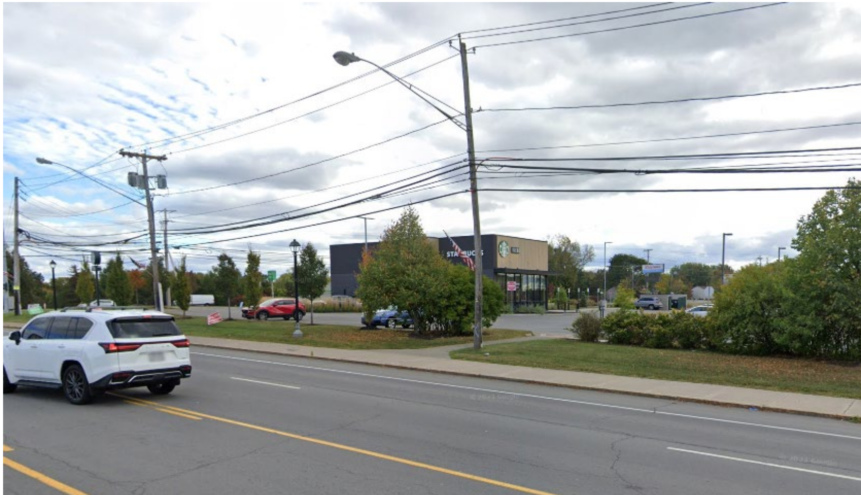
Pole in front Walgreens on Calkins Rd just West of E. Henrietta Rd
