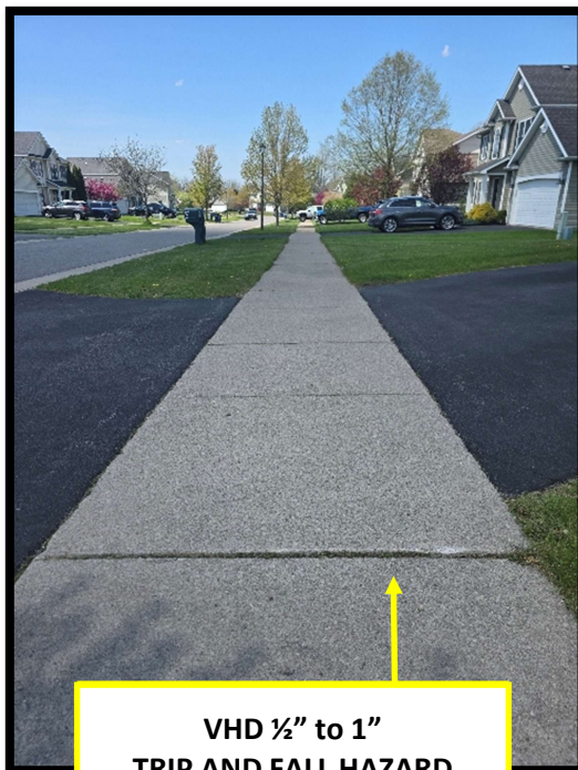
VHD ½" to 1" TRIP AND FALL HAZARD Repairable using Precision Concrete Cutting Process
