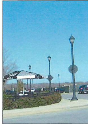
Figure 15: Example Light Pole and Fixture
