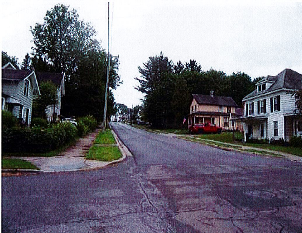
Barrett Street facing east
