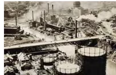
Source: Rochester City Hall Photo Lab
