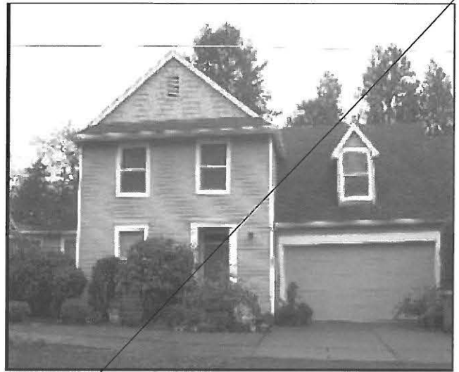
20th century construction in Old Town built to the vernacular style
