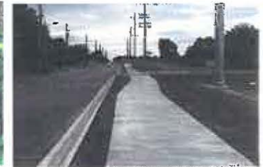
Shared Use Path in Roadway Right-of-Way
