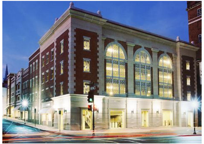
Attached liner building with exterior garage wall maintaining the architectural character of the rest of the structure.
