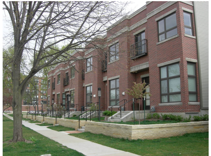
Elevated terrace to distance residential building from public sidewalk in urban residential area
