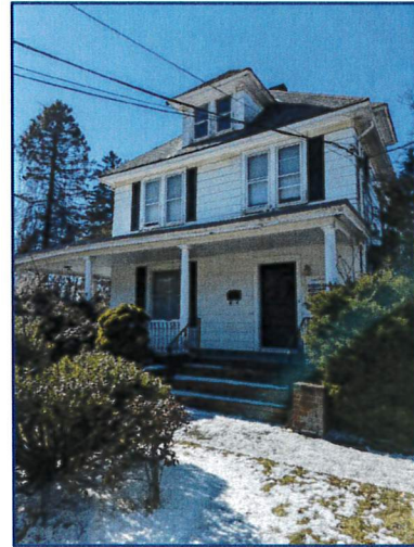
Photo 2 - Building on Lot 8
