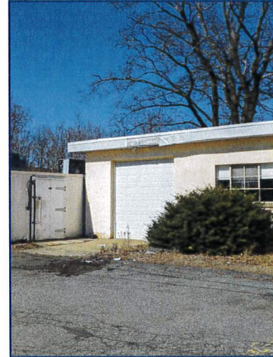
Photo 6 - Building on Lot 26
