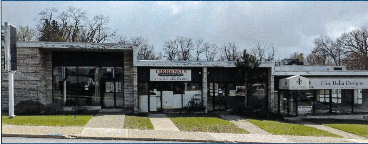
Photo 1 - Commercial building on Lot 1
