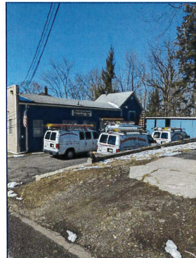
Photo 5 - Industrial building on Lot 19
