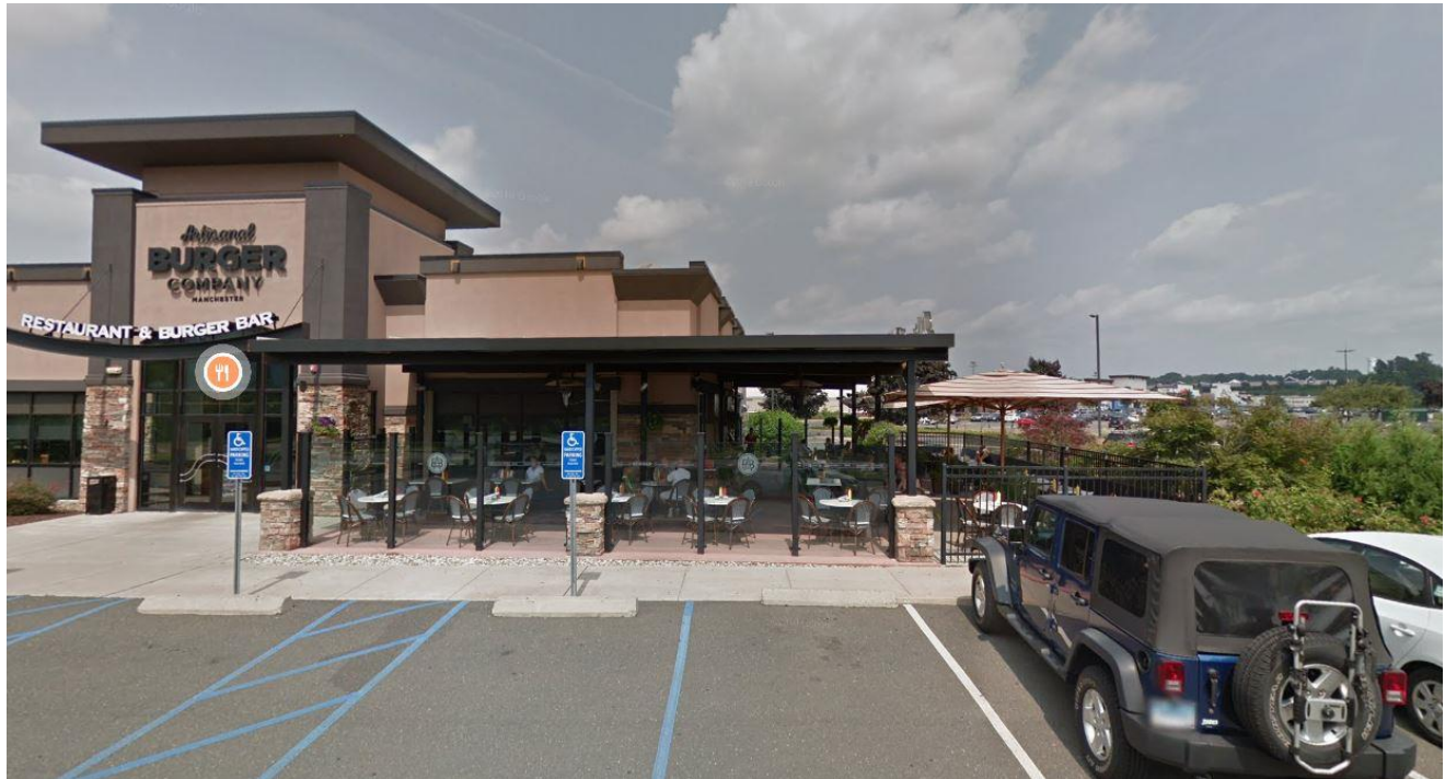
Existing Patio (Google Street View)
