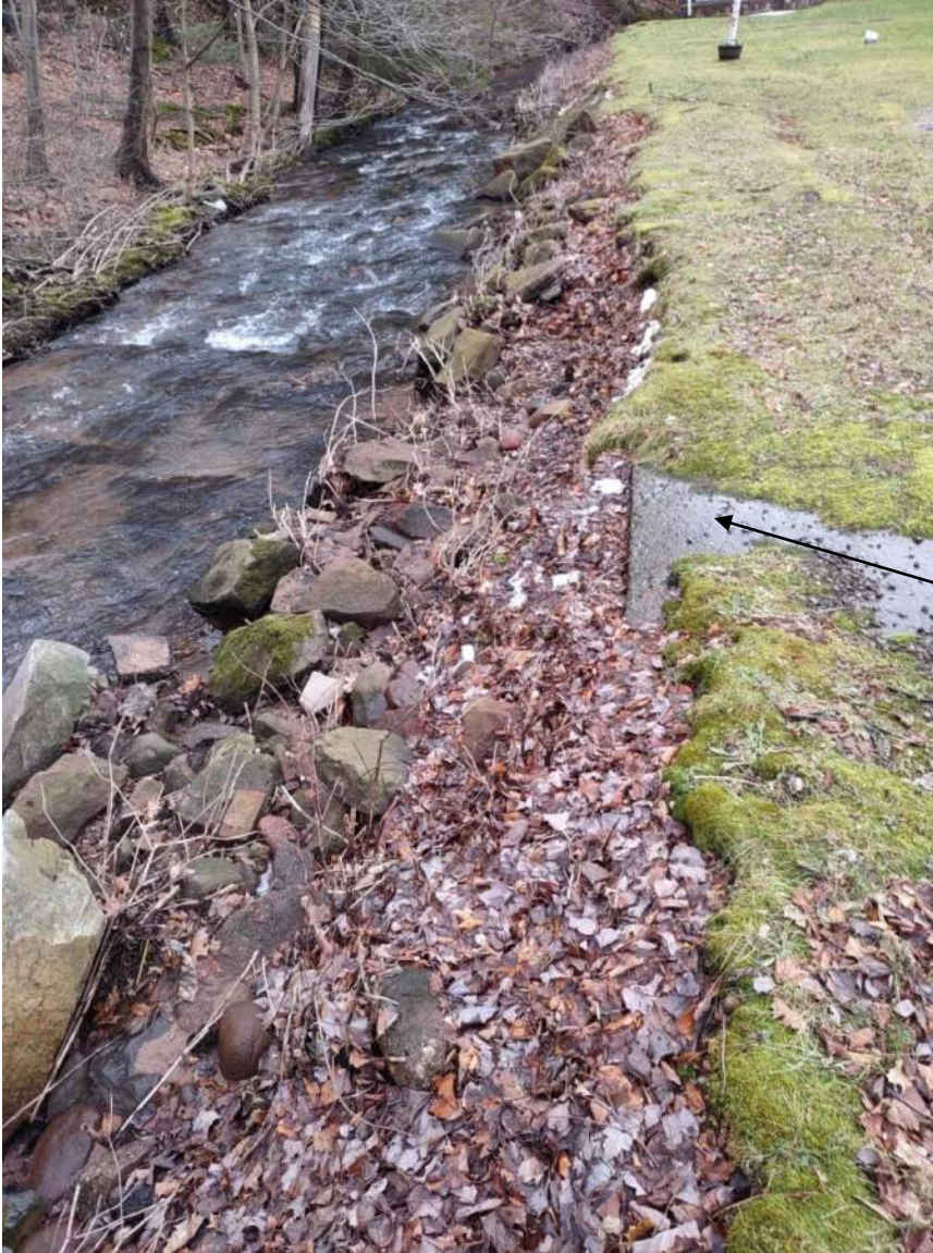
Scour near slab to be removed
