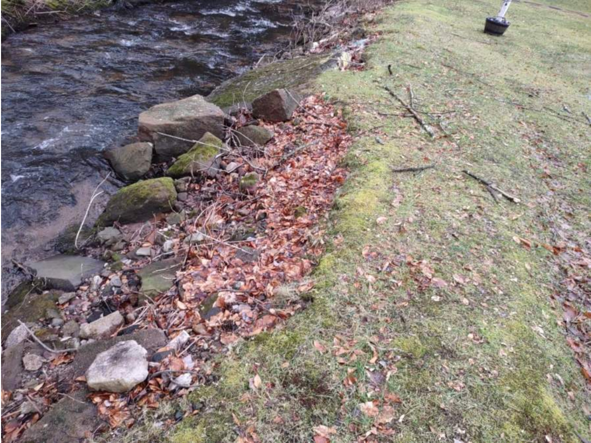
Nasty Scour- Since summer 2021, clean loose debris and armor with rip rap
