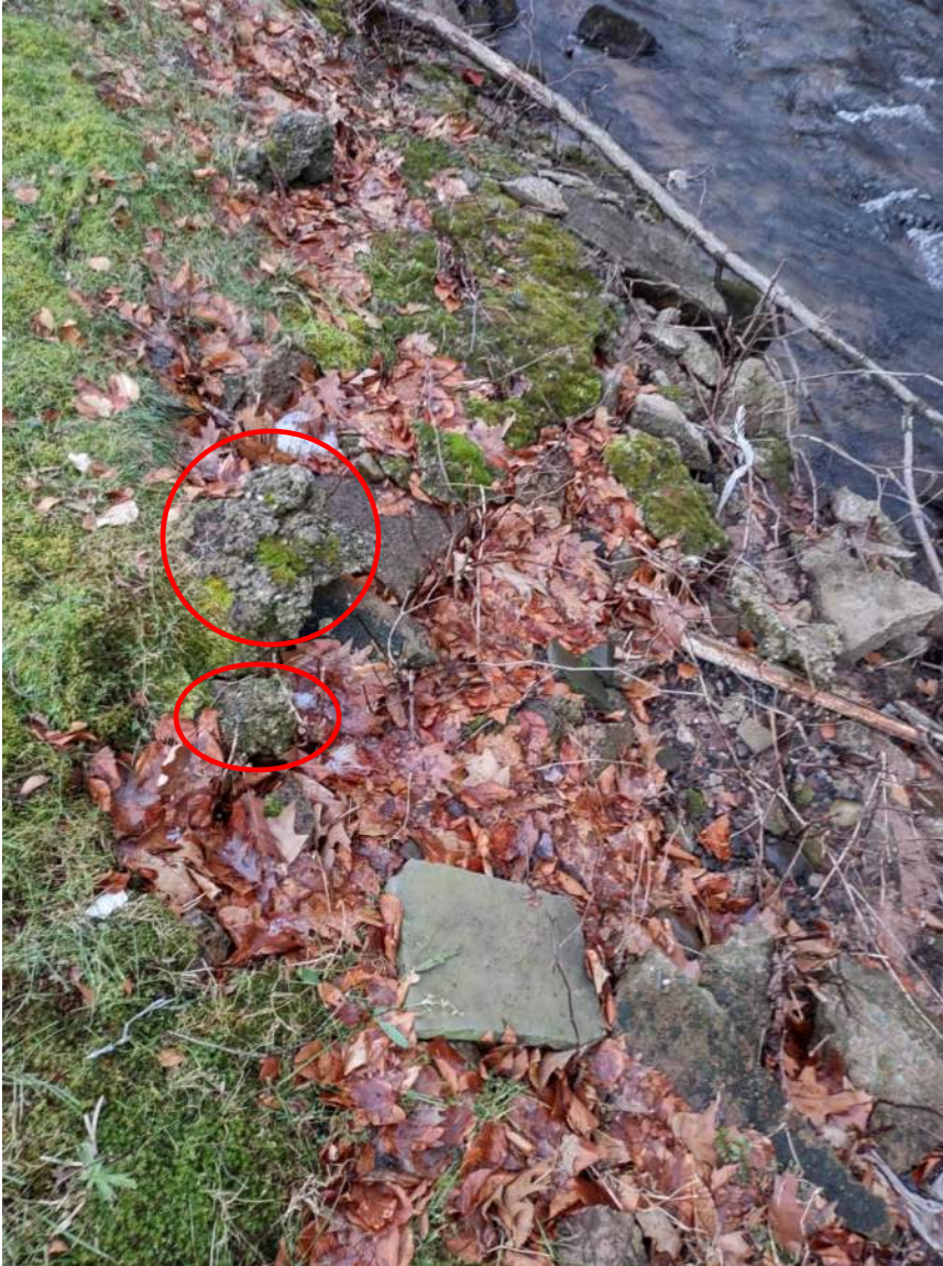
Concrete embedded in bank- Ugly but leave alone
