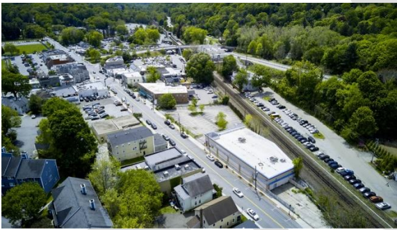
Existing Conditions View
