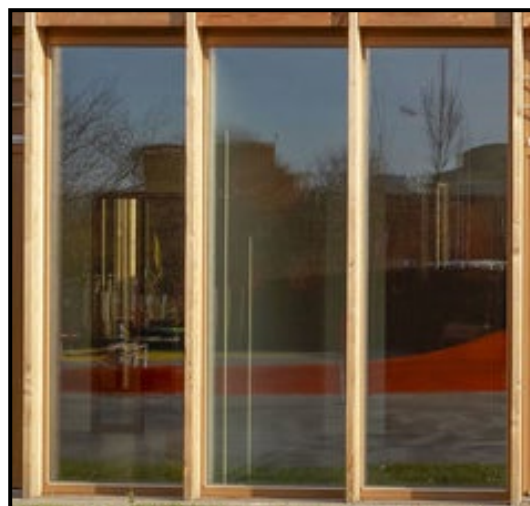
EXPOSED TIMBER STRUCTURE
