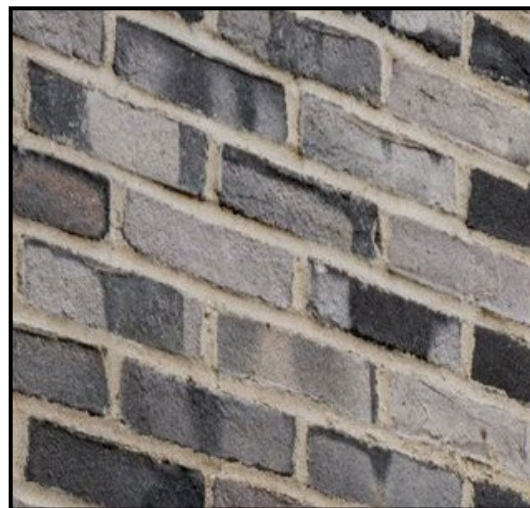
RUNNING BOND BRICK CLADDING
