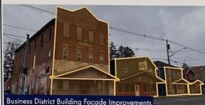
Business District Building Facade Improvements
