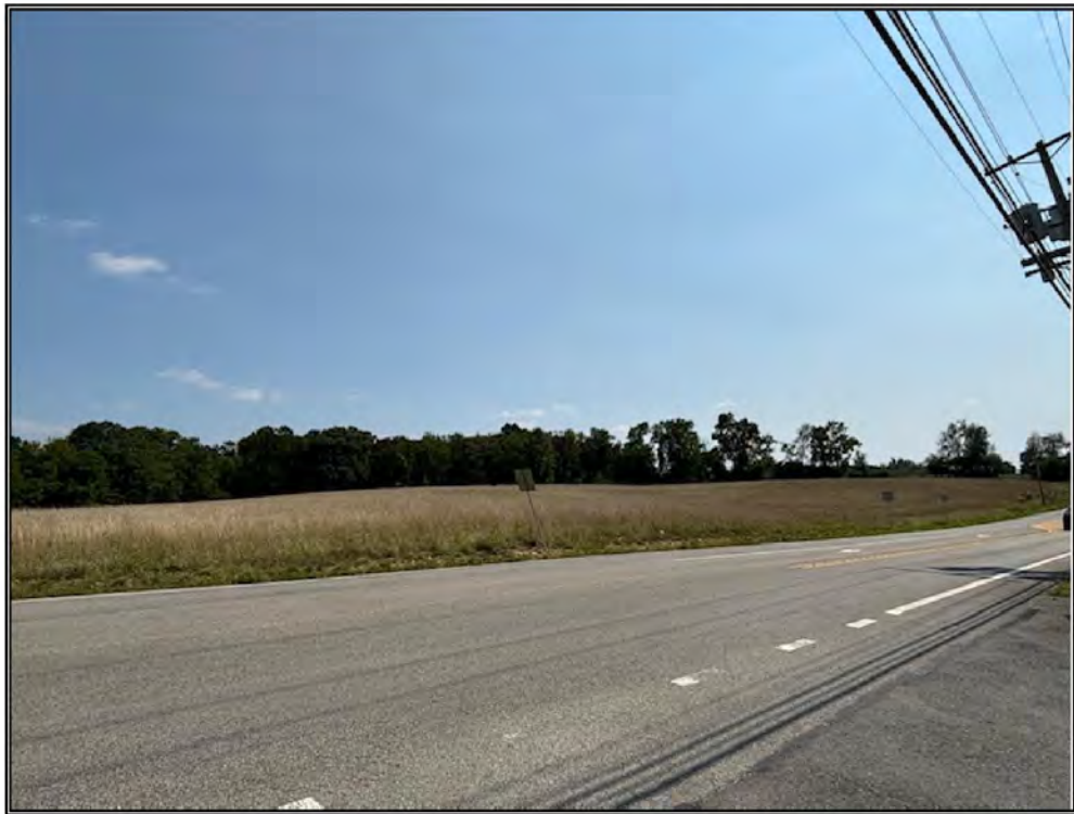
Babcock Boulevard and subject property
