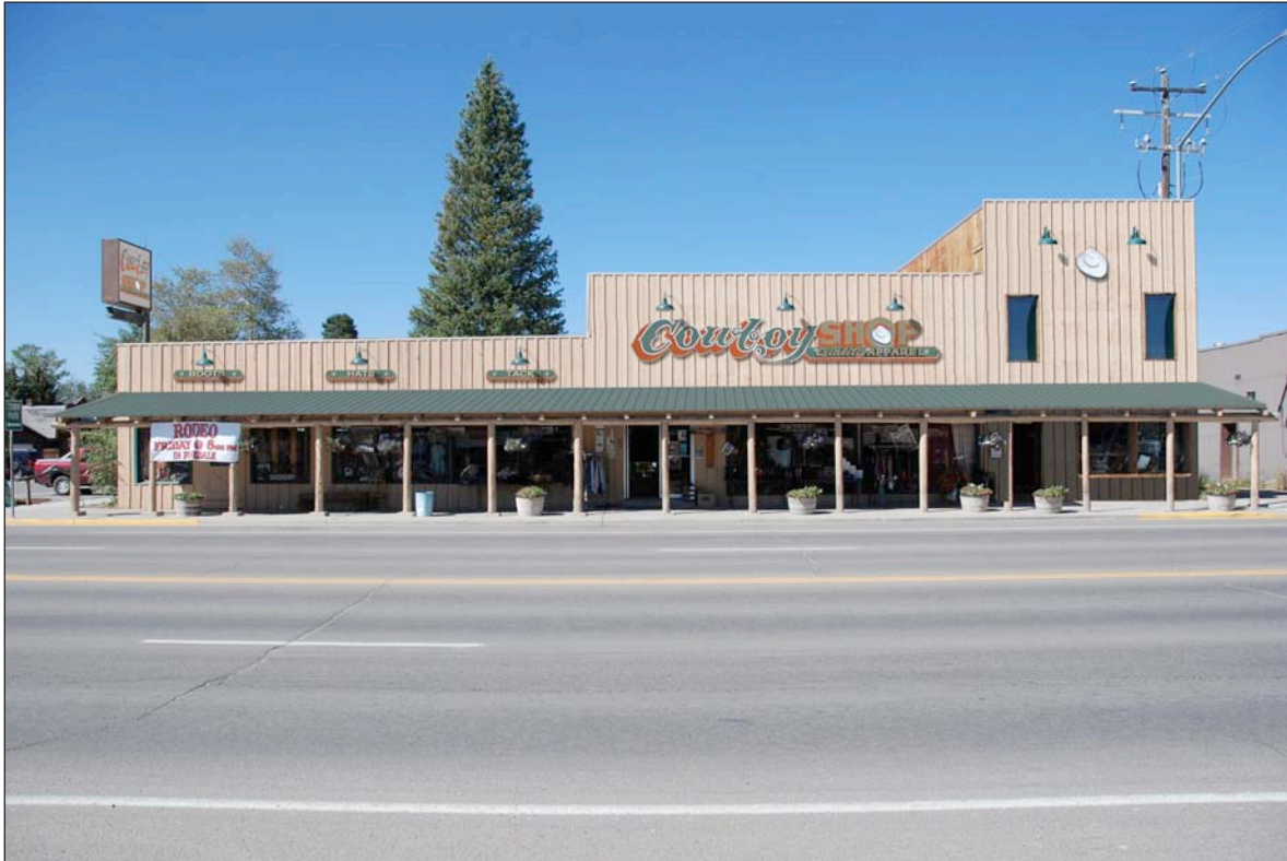
Figure 8: Proposed Conditions – In order to unify all three buildings and pay homage to the traditional American West Style of a simple false front, the rightmost building would receive a false front tall enough to conceal the angular nature of the roof. The middle building's false front would be raised to a height that splits the difference between the height of the left and right building parapet. This has the added benefit of providing a suitably scaled backdrop for their sign. Additional gooseneck lights and small signs and icons serve to promote the items for sale in the Cowboy Shop as well as to break up the monotony of the upper facade. Finally, the perpendicular sign panels are removed and replaced with signs that promote the Cowboy Shop.
