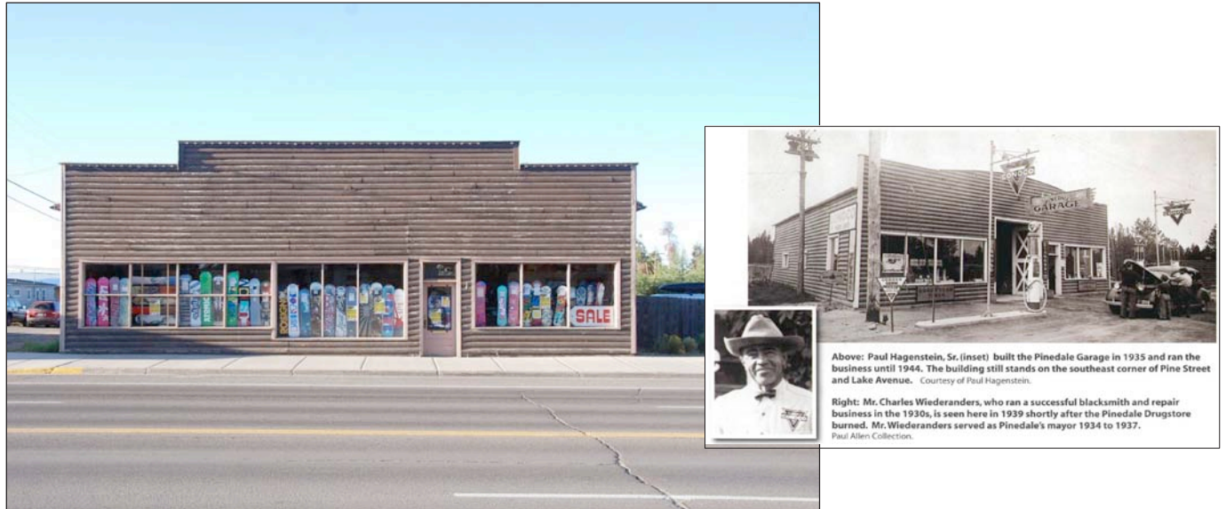
Figure 5: Existing Conditions – The current conditions reveal most of the original features of the building when it served as the Pinedale Garage (see inset historic photo) with the exception of the recessed entry bay. The upper facade lacks and detail to break up an otherwise large, blank wall. Finally, the building is in need of a fresh coat of paint or stain.
