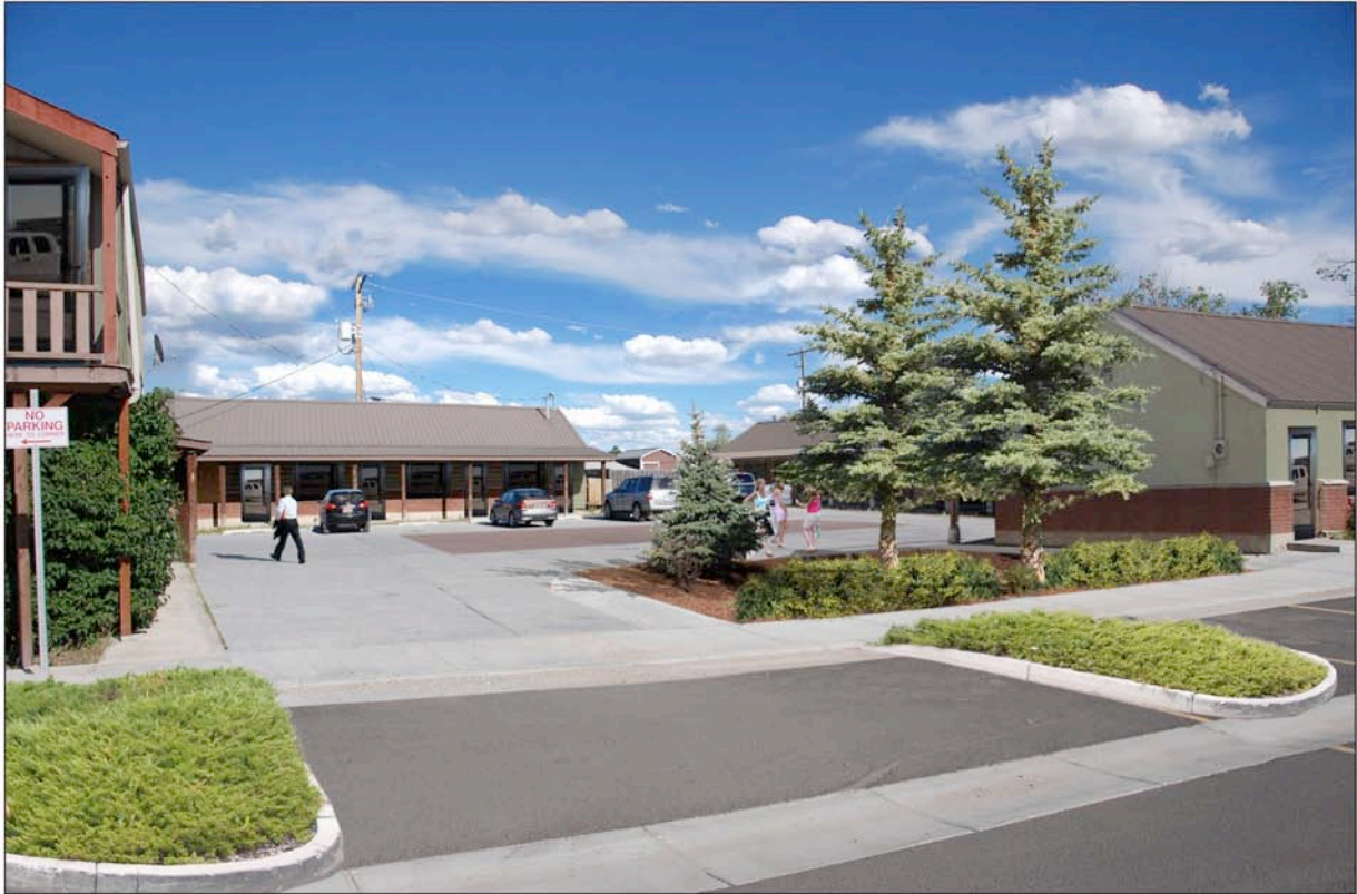
Figure 16: Proposed Conditions—The proposed redevelopment use for this site is a micro-enterprise retail site. The individual room configuration that makes them ideally suited for business start-up spaces. The parking court provides easy access to the offices for workers and visitors alike. The removal of the later addition provides visual access into the interior of the court. The conversion of this property from its previous motel use to an micro-retail use can be done at nominal costs due to the condition and layout of the existing structures. Moreover, this rehabilitation would maintain the essential form of the historic motor court maintaining its historic reference for years to come.
