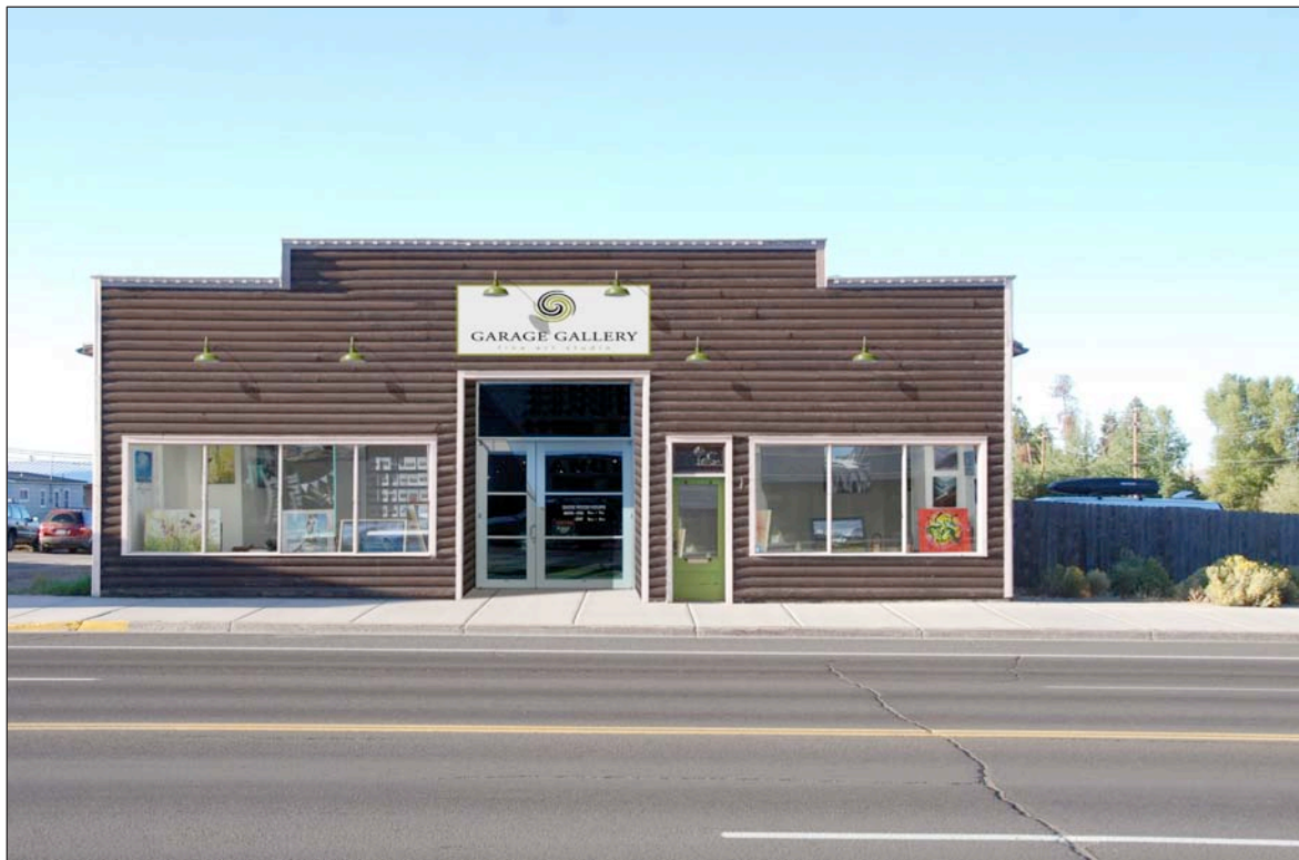
Figure 6: Proposed Conditions – Since the proposed adaptive reuse of this building is as a working art gallery/studio, reconfiguring the front facade to include the recessed entry as existed historically would prove beneficial for transferring large pieces of sculpture, paintings, etc. The addition of new signage and gooseneck light fixtures serve to break up the monotony of the upper facade. The proposed brand of the studio, “Garage Gallery,” recalls the historic use of the building.
