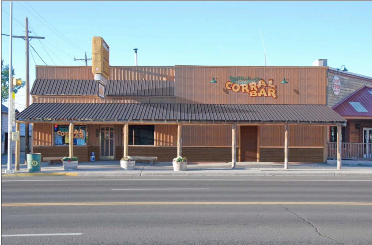
Figure 10: Proposed Conditions – By using a common siding and awning approach both buildings are unified visually. Also, by minimizing the signage, more attention is actually drawn to the signs that remain...one of which is a local landmark: the flashing neon sign of the "World Famous Corral Bar. The utilization of standing seam metal roofing on the awnings retains the form of the previous wood batten awning yet provides better weather resistance.
