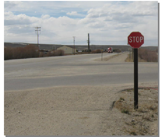
Figure 25 – Pinedale West Trail constructed with TEAS Funding
