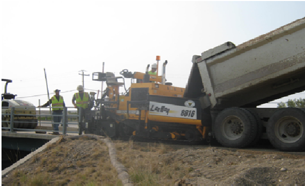
Figure 12 – Pathway Paving on Duck Creek Trail
