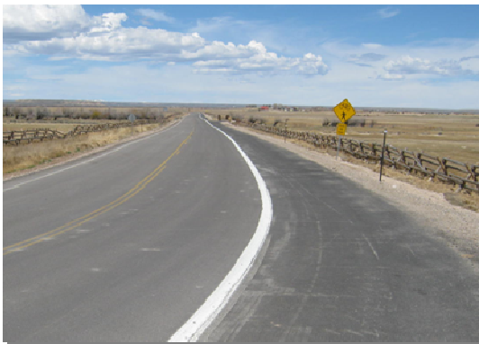
Figure 26 – Mickelson Lane Pathway constructed with Sublette County Funding
