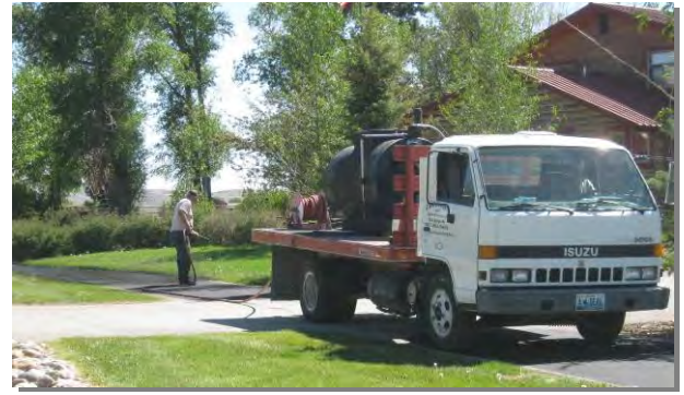
Figure 22 – Pathway Sealing along Willow Lake Road Trail
