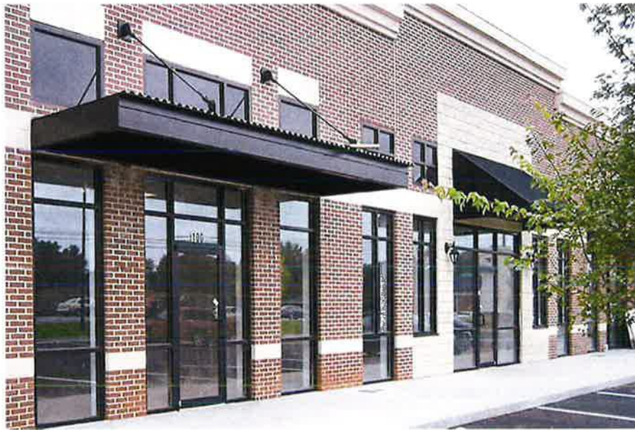
Figure 4 – Example architectural awning / canopy. (Source: preachtreeawnings.com )
