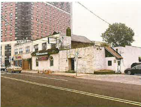
Block 4.04 (1349-53 Fulton St.) (6-7-23)
