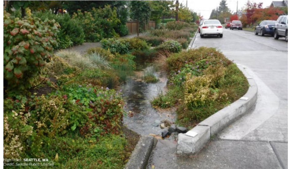
Image Source: Bio-retention swale, https://nacto.org https://ithaca.community/listings/cayuga-waterfront-trail-2/
