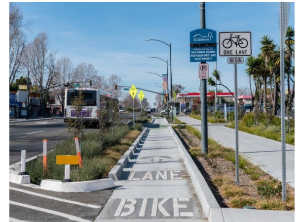
Image Source: Protected bike lane with rain, https://www.kneedeepitimes.org https://ithaca.community/listings/cayuga-
