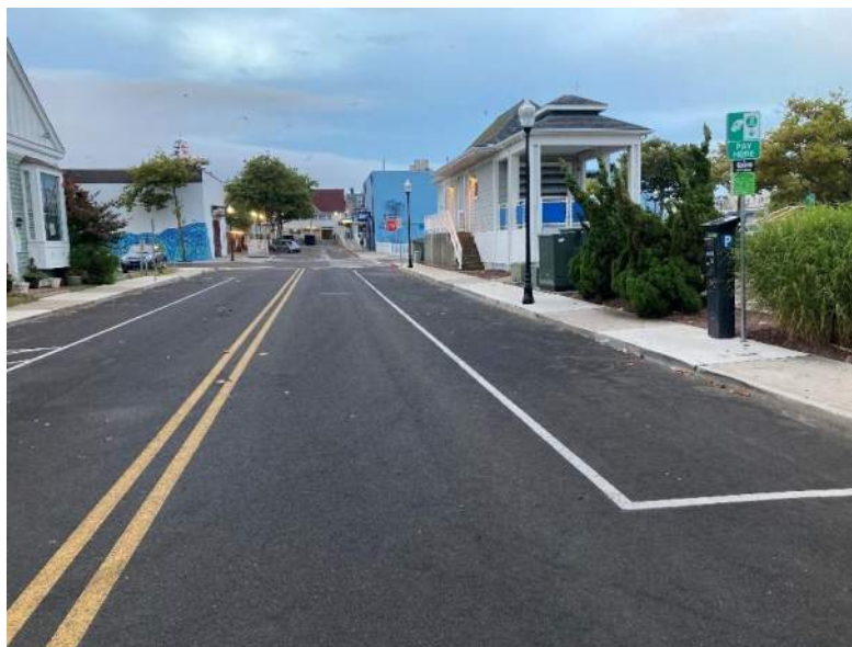
Figure 51: Example of Parking Delineation for a Specific Section of Road
