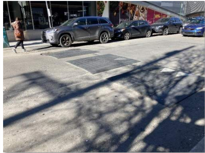
Figure 36: Temporary Speed Cushions
