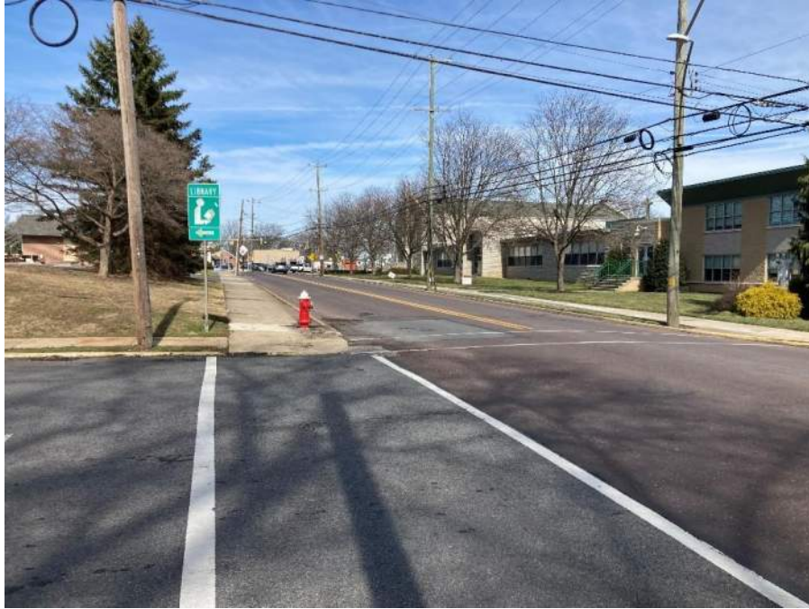
Figure 26: Uncontrolled Intersection of Washington Street and Lewis Road
