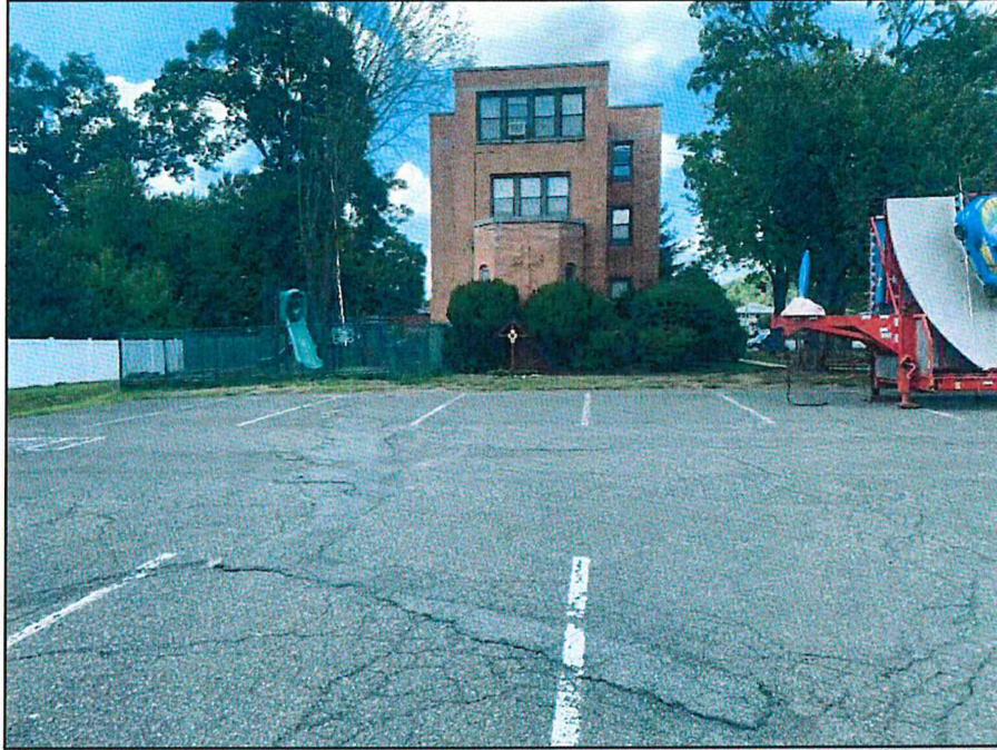
Image 3: Side View of Fatima House Convent facing Westfield Avenue
