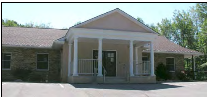
Penn Forest Township Building
