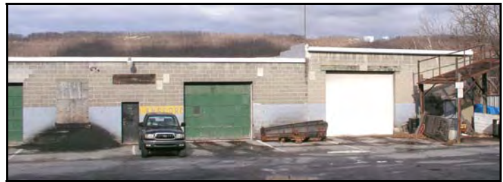
Lansford Street Department
