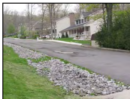
Stabilized Drainage Swale
