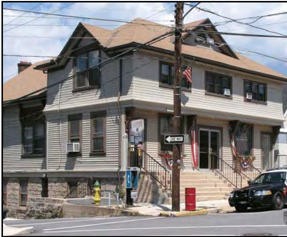
Lansford Community Center and Police Department
