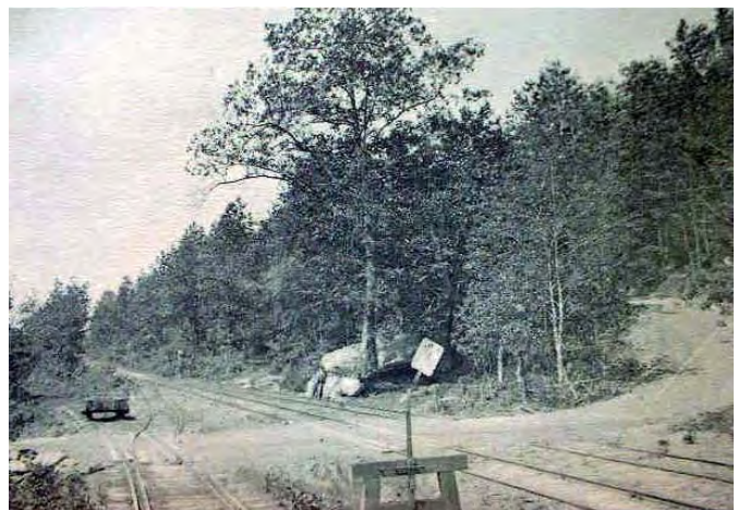
Switchback Gravity Railroad in the area of the crossover. (photo: www.Summit-Hill.com )
