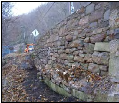
Jim Thorpe Retaining Wall
