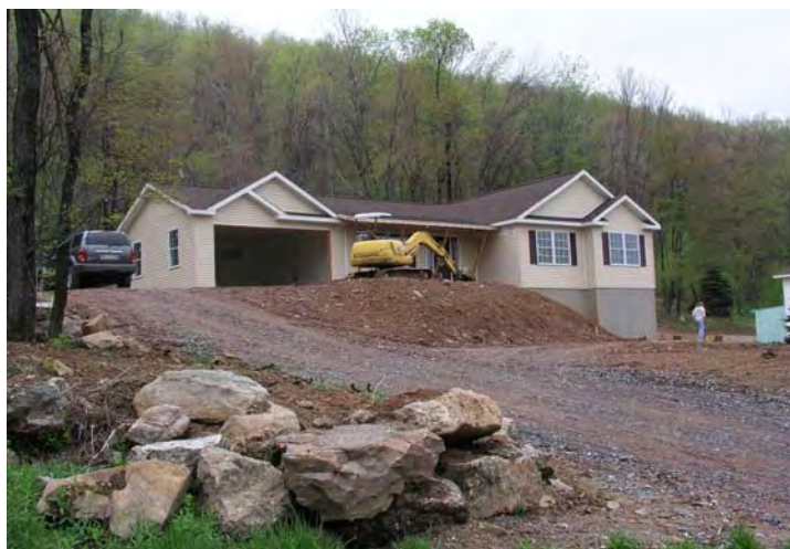
New home construction.
