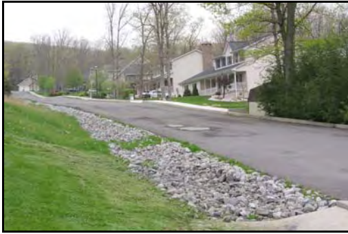
Stormwater Swale, Jim Thorpe
