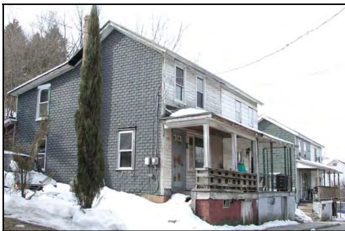
Repairs Needed, Lansford
