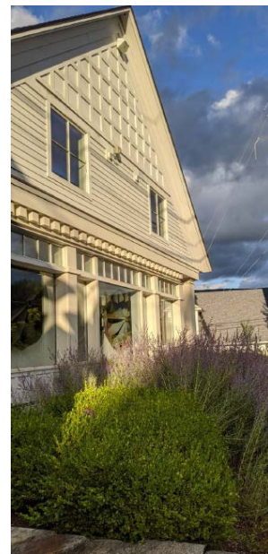
Figure 11. This is an example of facade windows that meet the design standards for the TC District.
