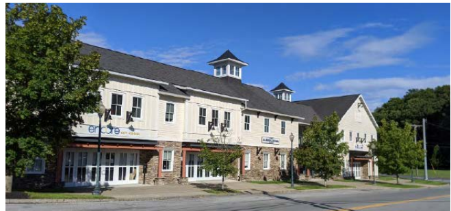
Figure 8. Example of a new building showing a roof design with cupolas consistent with the rural character in Union Vale. This also shows appropriate facade breaks used to improve the aesthetics of a large building.
