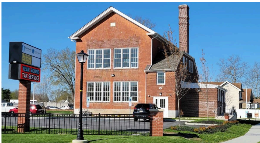
Renovated McCay Avenue Schoolhouse
