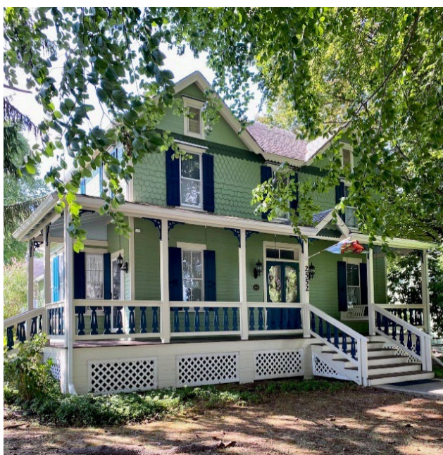
Renovated 2552 Central Avenue
