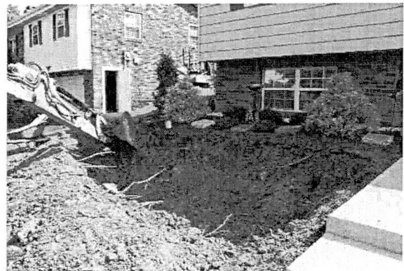
Excavate rain garden at least 10' from foundation
