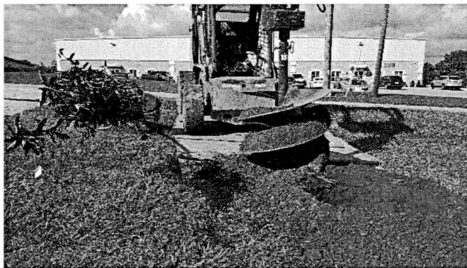
Plywood sheets protect lawn from compaction
